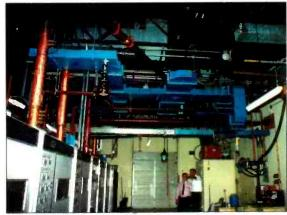
A combiner network using waveguide is common in UHF transmitter installations.
