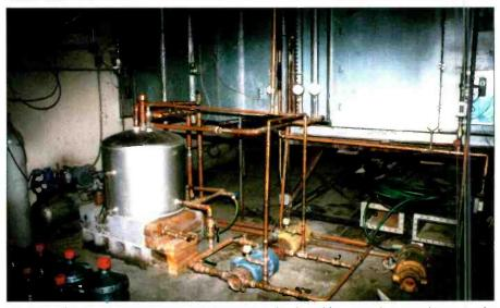
A portion of the heat exchanger along with the pumps and tank used for a water/vapor cooling system for klystrons. (Photos courtesy of David Birdsong, KSMO-TV.)
